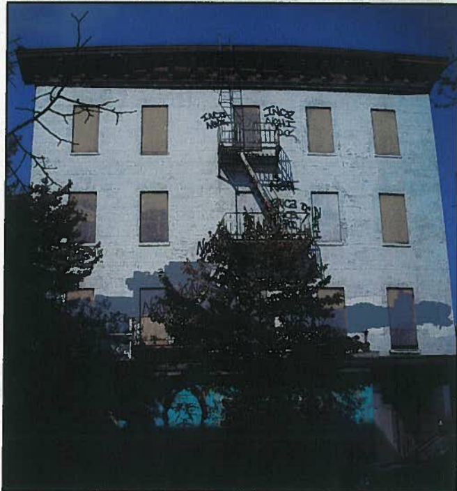
The current view of the Franklin Street façade.
